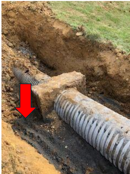
Photograph No. 2 – View of the initial excavation exposing the existing pipe and anti-seep collar. The edge of the section of the pipe sitting over the concrete pad is noted with arrow.
