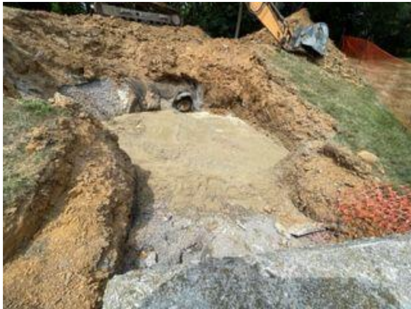
Photograph No. 10 – Additional view of flowable fill on July 8, 2024, facing north.
