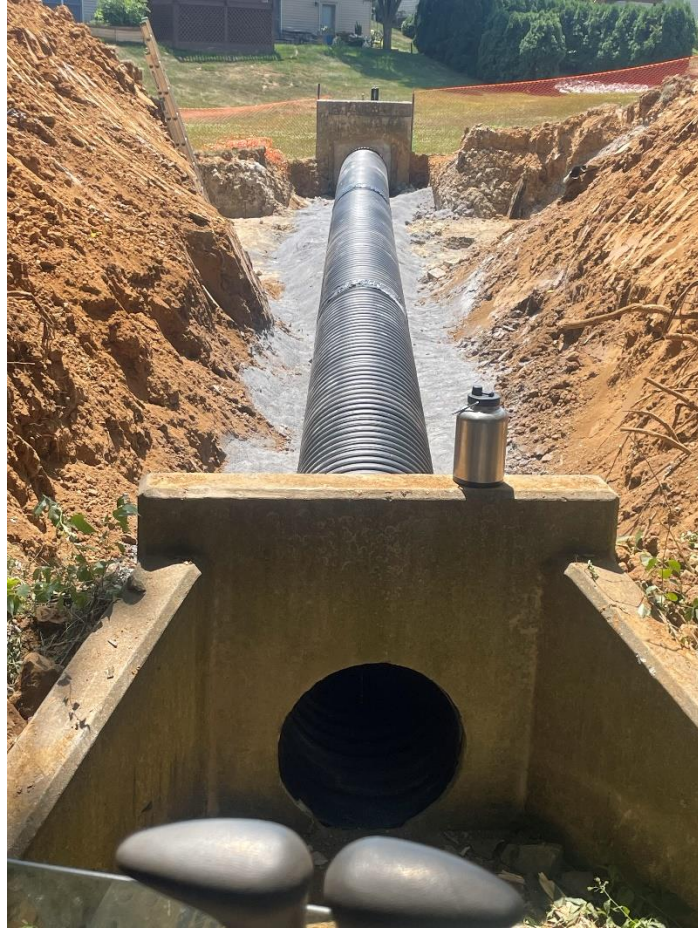
Photograph No. 17 – New 24-inch pipe after placement
