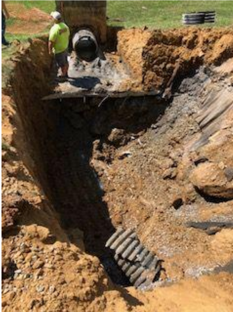
Photograph No. 6 – View of excavation as cleanup of soft/wet subgrade continued.
