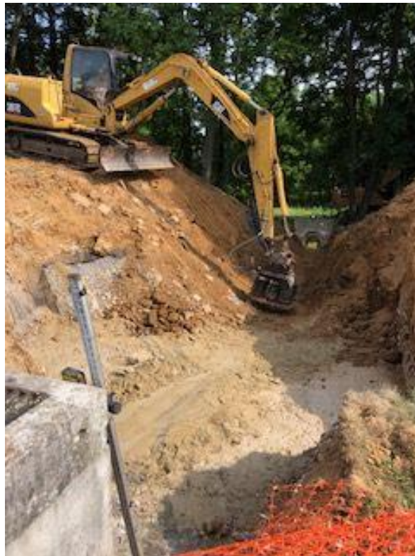
Photograph No. 16 – Contractor compacting subgrade
