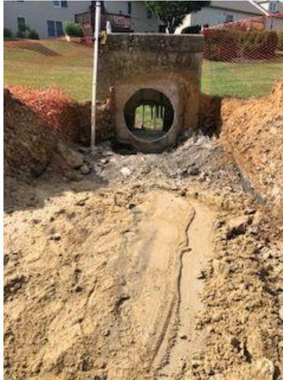
Photograph No. 11 – Photograph on July 9, 2024 after flowable fill placement of July 8, 2024
