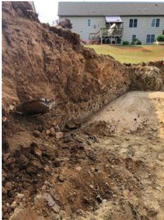
Photograph No. 12 – View of flowable fill along eastern sidewall, facing south
