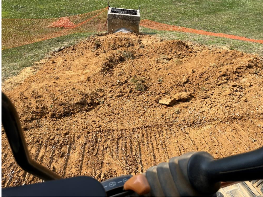
Photograph No. 19 – Grading/backfill activities near the outlet structure
