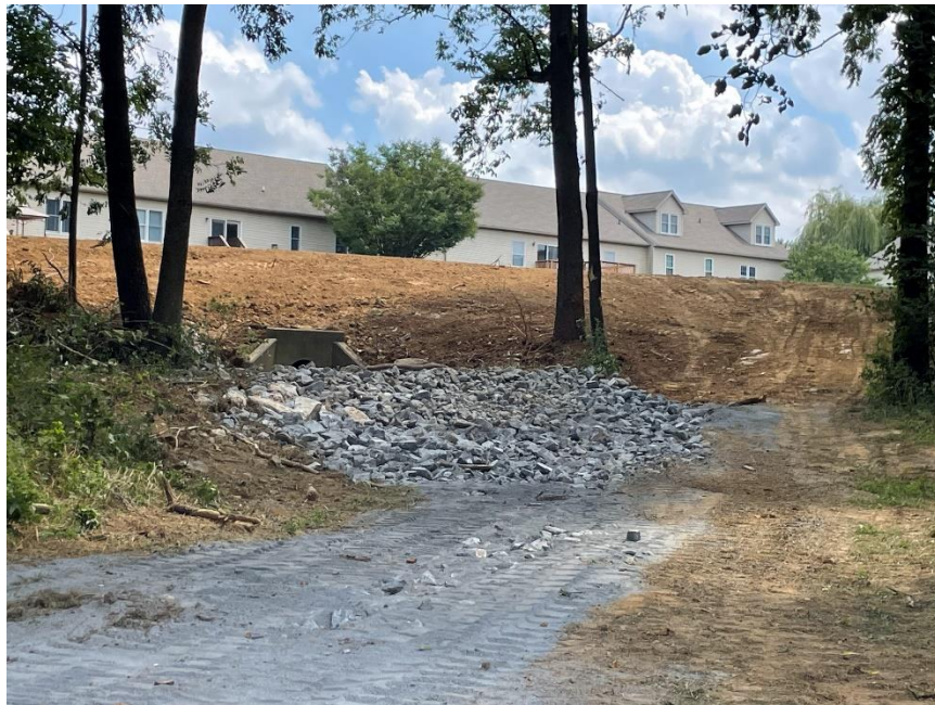
Photograph No. 20 – Completed backfilling/restoration at end wall on July 10, 2024
