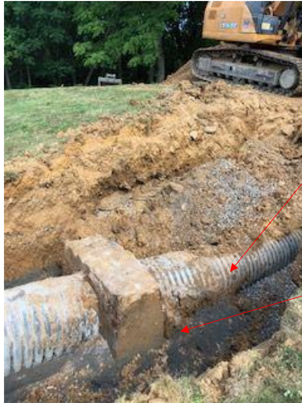
Photograph No. 3 – Additional view of exposed pipe facing northwest. Arrow notes the section of pipe that was obviously damaged and leaking.
