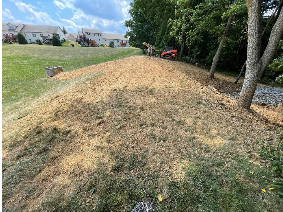
Photograph No. 21 – View of restoration across top of berm, facing west
