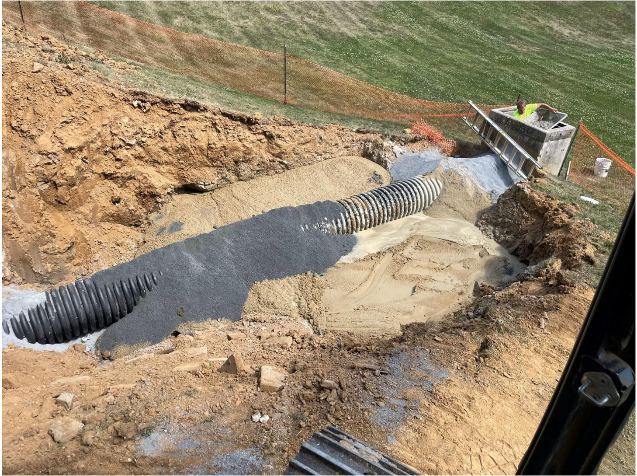
Photograph No. 18 – Additional flowable fill and backfilling placement around new pipe
